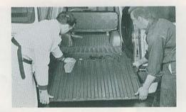
Remove ten screws, and with a little help, you can lift the heavy engine compartment lid . . .
