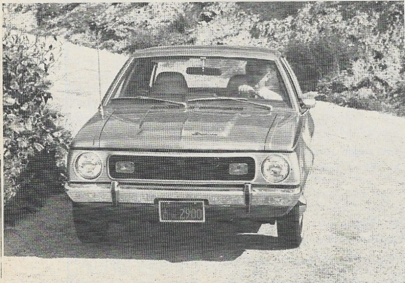
C. Like the Hornet, the Gremlin grille is a plastic composition and bumpers are shared. Special feature of all AMC headlights is a filament that glows after burn-out.
