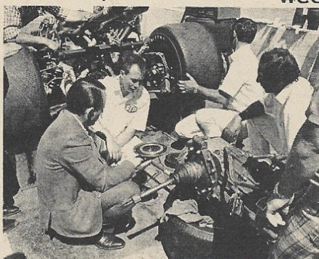
A slipping clutch forced Mario Andretti's crew to pull the transaxle just 45 minutes before start of race.
