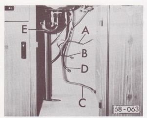
remove fuse in in-line fuse holder for water pump, disconnect hot wire (A) and ground wire (B) from fuse box, gas range connection (C) and city water hook-up (D) (E = sink drain pipe)
