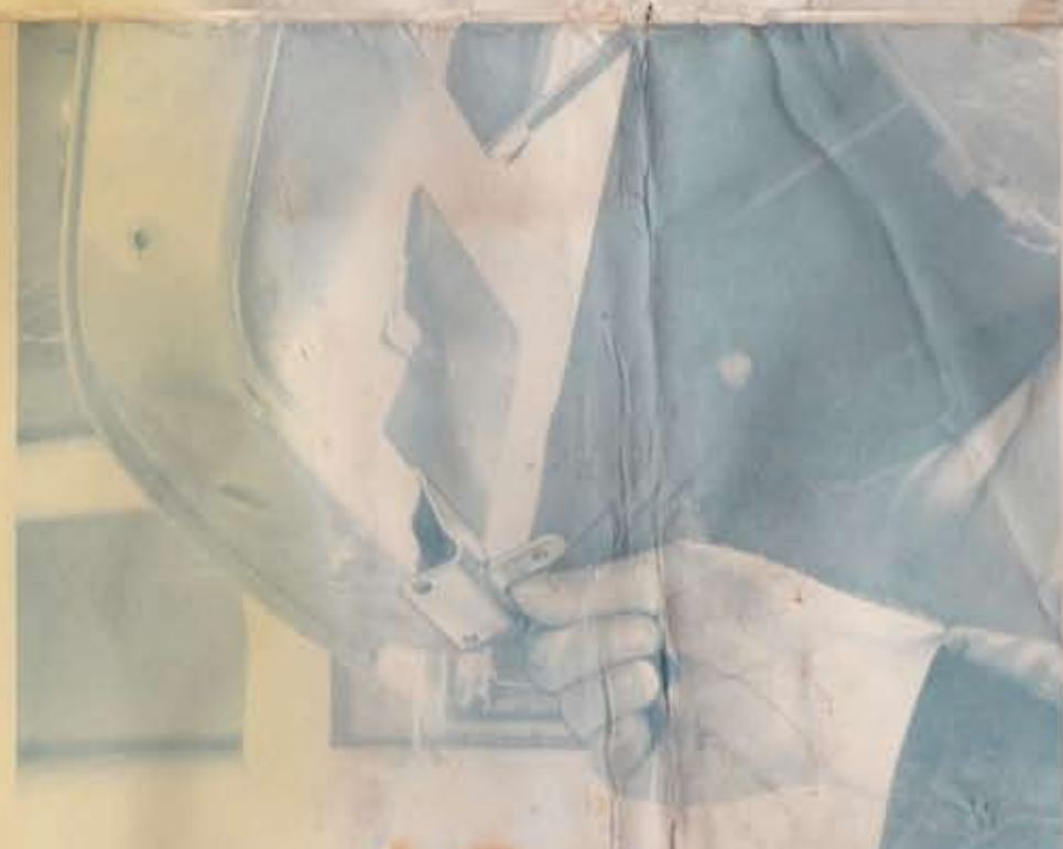
6 Lift door-panel, set the door bracket into the cut-out at the base of the door, as close as possible to the front of the door. Pull catch down and drill 3/16" holes from underneath. Insert 3/16" bolts with lock washers and nuts.
