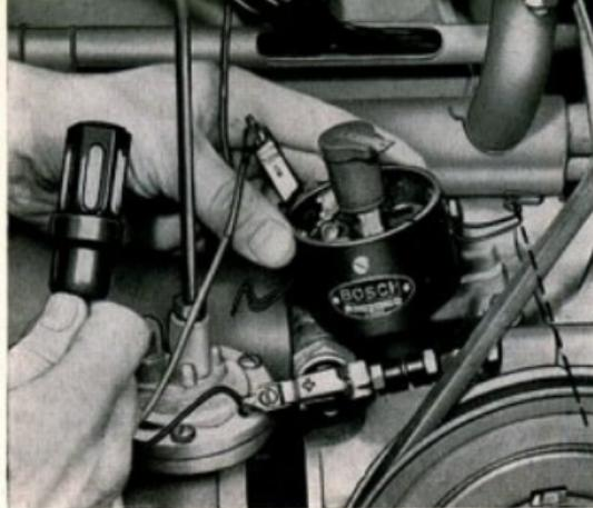
for firing on the No. 1 cylinder (see mark on rim of distributor base). Loosen the lock screw below the distributor base and rotate the distributor body clockwise until the contact points are closed. Now switch on the ignition and rotate the distributor slowly anti-clockwise until the contact points just start to open. This may be seen and heard, for a spark will jump from one point to the other.
