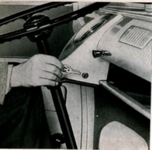
The ignition key starting enables you to start the engine by merely turning the ignition key. First the ignition is switched on by turning the key to the right. The red generator warning light and the green light for the oil pressure will light up. To start the engine, the key is pressed against a spring load and further turned clockwise until the starting motor operates. As soon as the engine fires, release pressure on key to disconnect starting motor.
