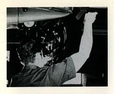
Now, pull down on the handle of the checking lever. This expands the torsion arms and reveals any ball joint play.
