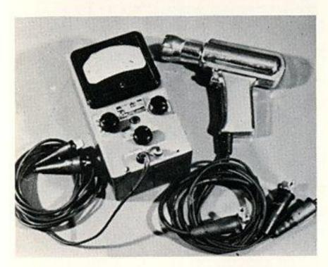
For this operation, a stroboscopic timing light and a tachometer are essential.
