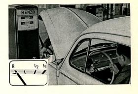
21/12 We remove the protection panel behind the instrument panel. With the help of a screwdriver we turn the slotted knurled nut and set the fuel gauge needle on the line R. A helper will have to observe the gauge during this operation. The next picture will show you how to check the fuel gauge when the tank contains an unknown quantity of fuel.
