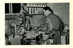
21/7 We have already seen that electronic devices are used by the inspectors to identify even the smallest deviation on the recordings. On the final assembly line the torque wrench is usually used for checking the tightness of important connections on the frame. The man you see here is checking whether the brake line nuts are tightened as prescribed to between 1.5 and 2.0 mkg (11 and 14 ft. lbs.).
