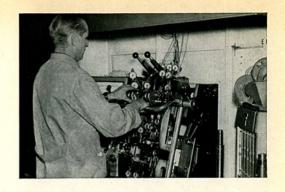
21/6 Here we see one of the 34 recording cabins for the transmissions in the Cassel plant. As shown here, each transmission is checked functionally and for silent operation before it is sent to Wolfsburg or Hanover. The inspector's trained ear is helped by a microphone which transmits the oscillation frequencies electronically to the recording instruments. Here you see the microphone above the transmission case.
