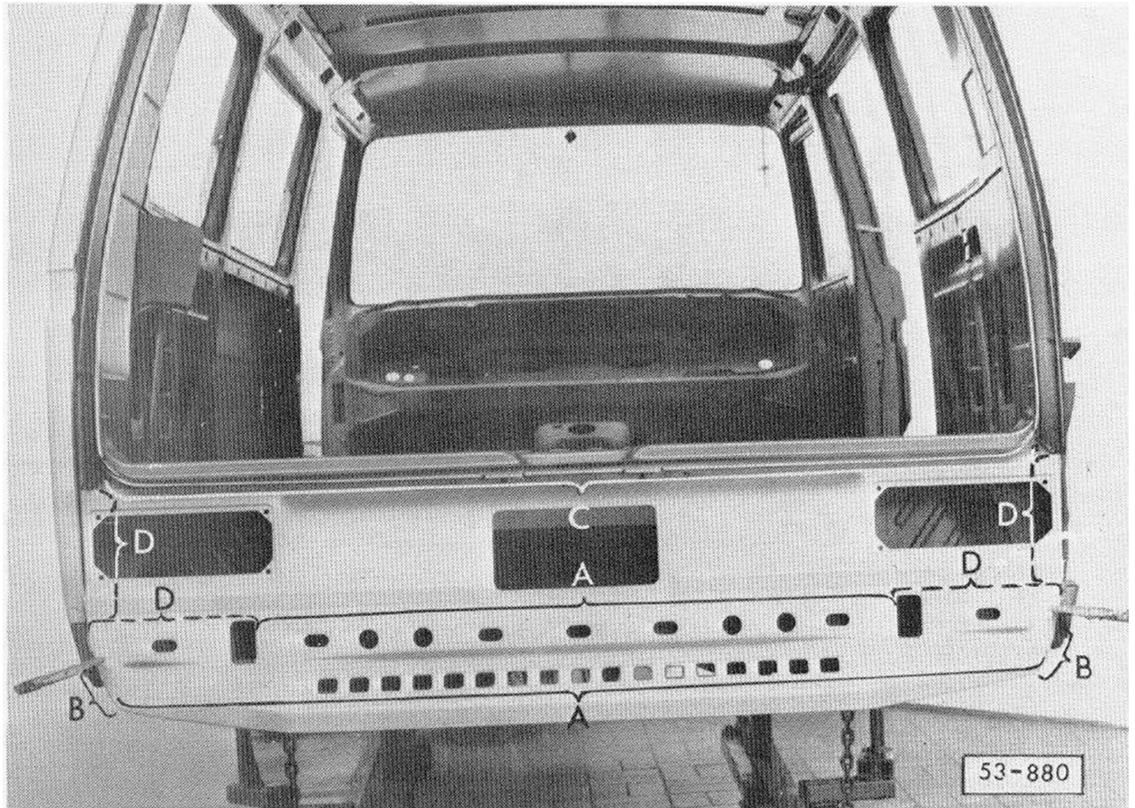
Fig. 3: Aligning and welding in rear apron
