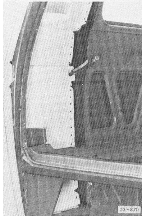
Fig. 10: Aligning corner panel
